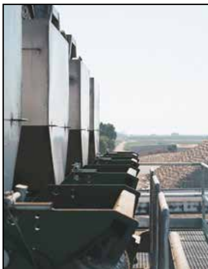
Vierra Dairy is operated with a wide range of new technology to improve efficiency, increase cow comfort and reduce carbon footprint, including this methane digester installed in August 2020.
